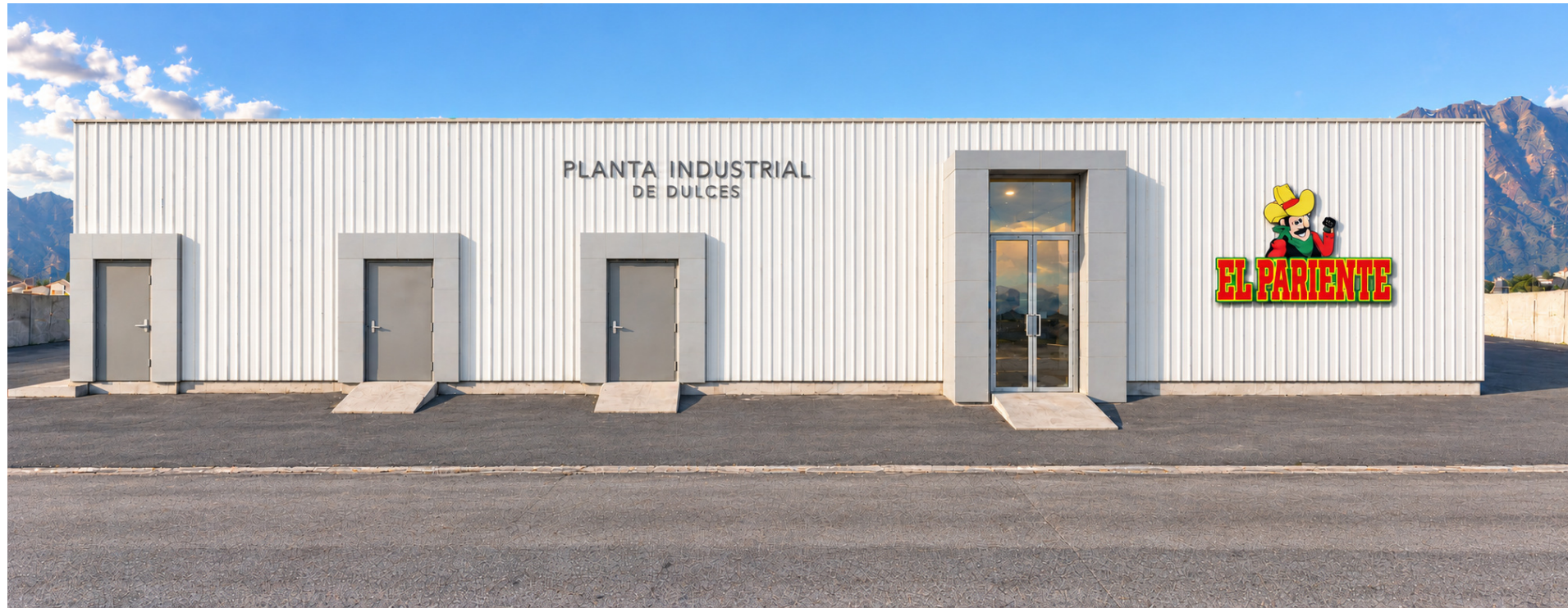
a East facade · main entrance and service openings
